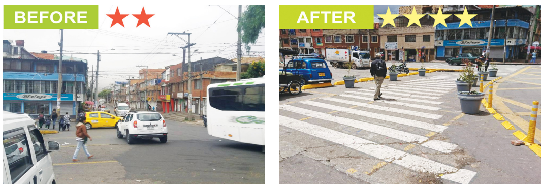
Figure 44. SR4S assessment results before and after infrastructure modification
